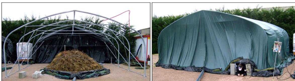
Figure 3. Photographs of the storage greenhouse, uncovered (left) and covered (right).
