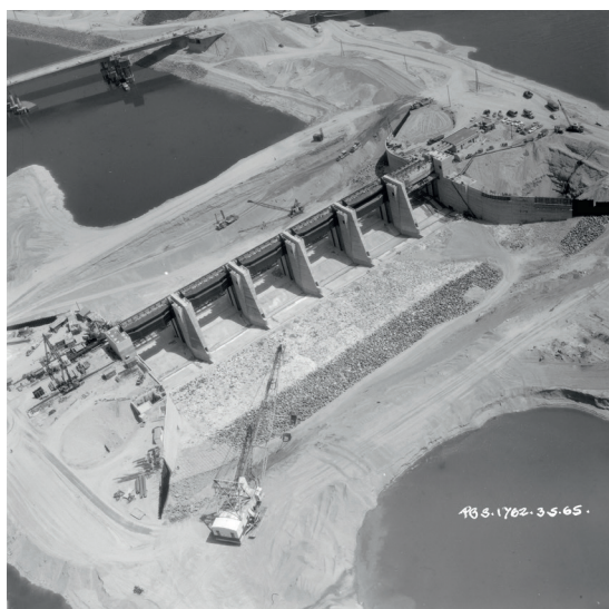
Figure 8.7 – Barrage de Pierre-Bénite / © CNR
