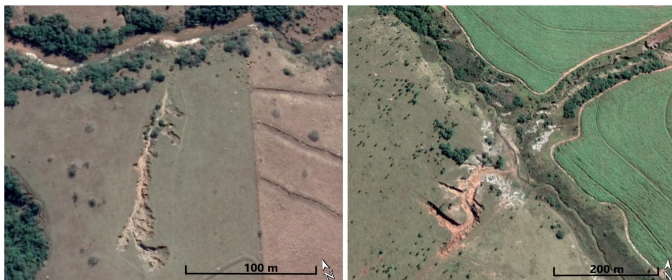
Figure 11. Gully erosion in the eastern parts of the study area.
