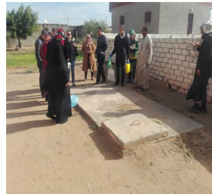
No wastewater treatment system
