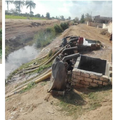
High salt concentration of the ground water and canal irrigation
