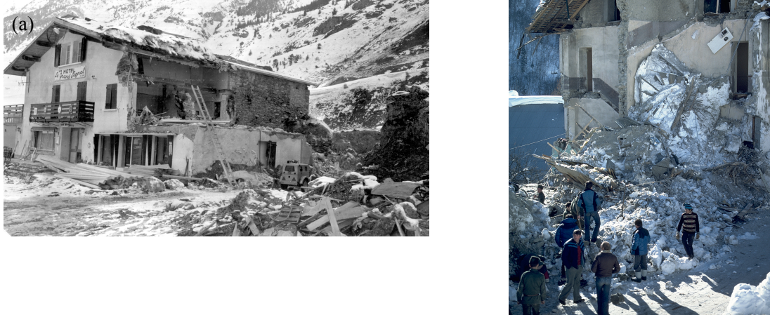
Figure 1: Examples of damage caused by snow avalanches to residential buildings in the Maurienne valley located in the French Alps: (a) on February 24, 1970, in Lanslevillard, Savoie, France (Photo credits: ©Section d'étude des troupes de Montagne, Chef de Bataillon Talon (1970)); (b) on January 20, 1981, in Saint-Colomban-des-Villards, Savoie, France (Photo credits: ©François Valla/INRAE).
