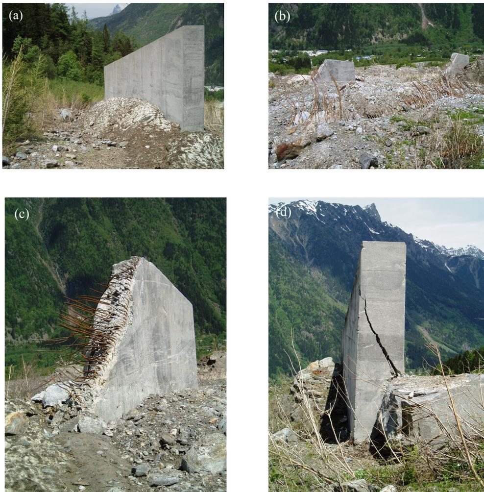
Figure 2: Overview of damage caused by a snow avalanche to different elements of the Tacconnaz reinforced concrete structure during the winter of 2005/2006. Damage intensity is sorted in four states: (a) without damage; (b) fully destroyed; (c) partially destroyed; (d) with cracks (Photo credits: ©François Rapin/INRAE).
