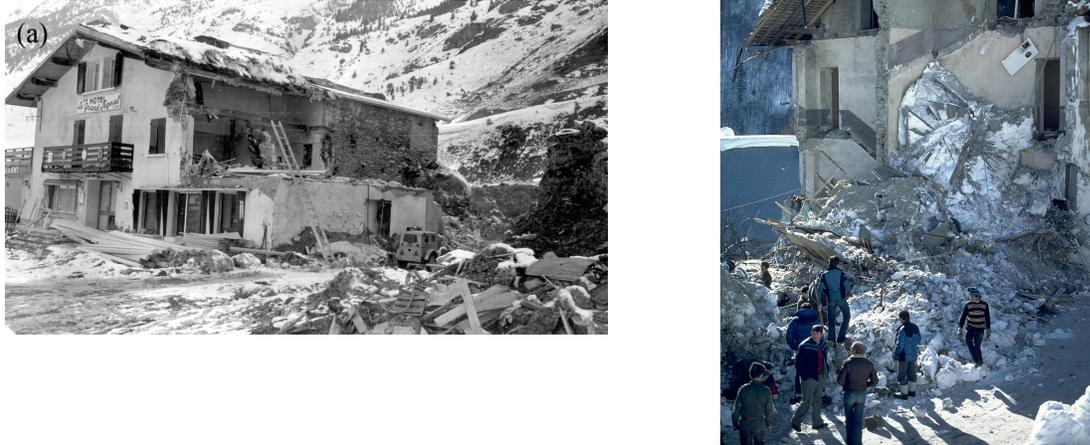
Figure 1: Examples of damage caused by snow avalanches to residential buildings in the Maurienne valley located in the French Alps: (a) on February 24, 1970, in Lanslevillard, Savoie, France (Photo credits: ©Section d'étude des troupes de Montagne, Chef de Bataillon Talon (1970)); (b) on January 20, 1981, in Saint-Colomban-des-Villard, Savoie, France (Photo credits: ©François Valla/INRAE).
