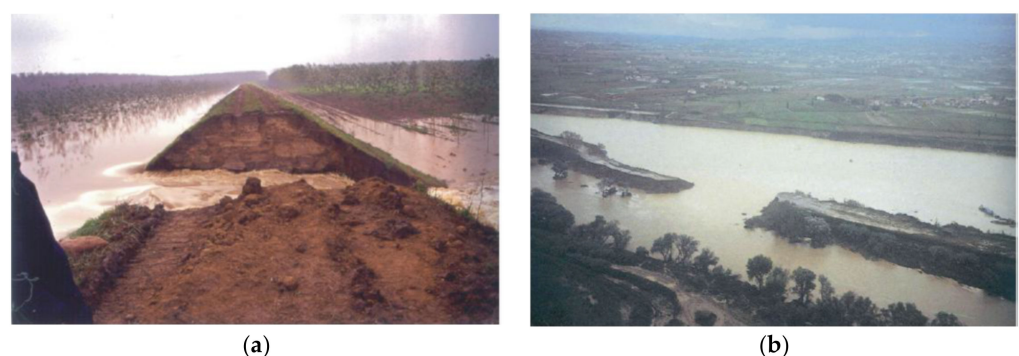
Figure 5. Examples of failure of: (a) the dyke of river Po in Mantova province (Northern Italy) during the flood event of October 2000, and (b) the dyke of river Arno in Tuscany (Italy) during the flood event of October 1992 (adapted from [17]).
