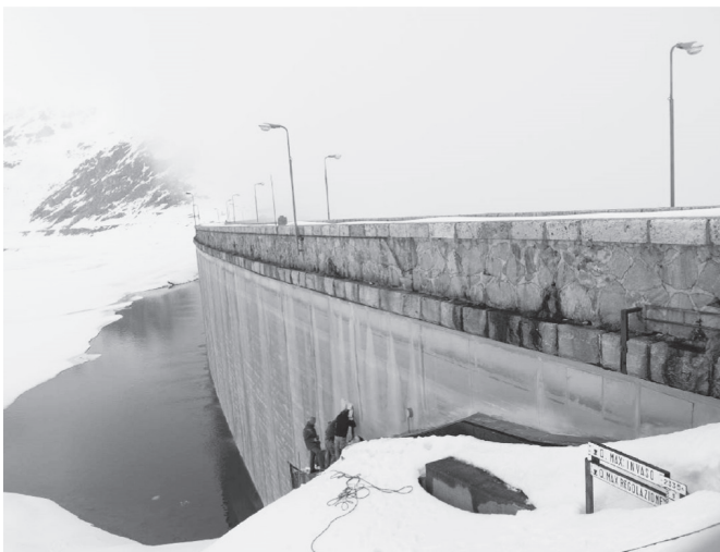
Fig. 4 - Camposecco dam samplings in Italy, courtesy D. Cazzuffi.
