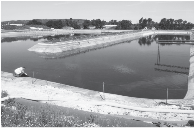
Fig. 3 - Pond lined with bituminous geomembranes at the Bazancourt sugar refinery at the time of geomembrane sampling for durability study (Touze-Foltz et al., 2015).
