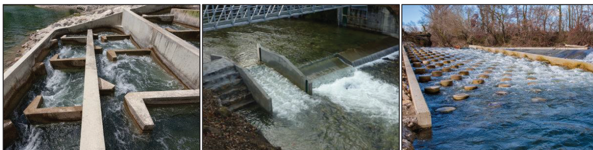
Figure 4: Examples of fishways; from left to right: pool-type fishway, baffle fishway, nature-like fishpass (credit: Sylvain Richard, OFB)
