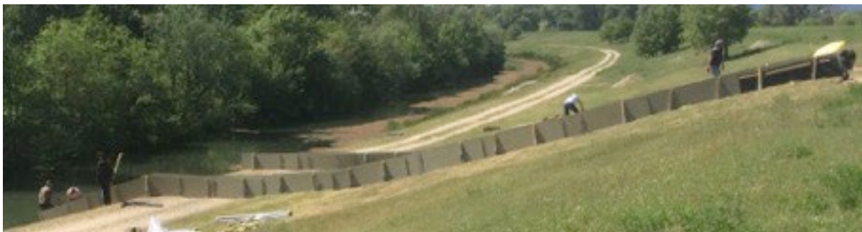
Figure 3. View of the two test channels. Channel 1 is in the foreground.
