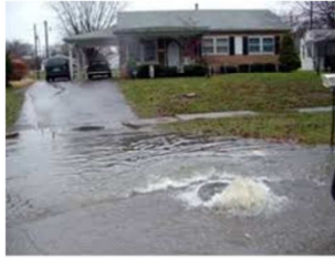
Sanitary sewer manhole overflow
