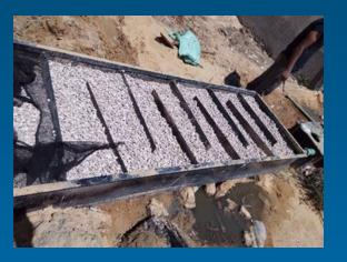
The flow cross-section and hydraulic gradient defined in the linear bio-filter must be maintained in the compact bio-filter. The possible width of the bio-filter depends on the space available laterally.
