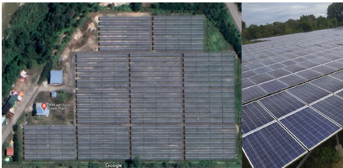
Figure 6. Snapshots of 2MWp Puchong solar farm in Selangor.
