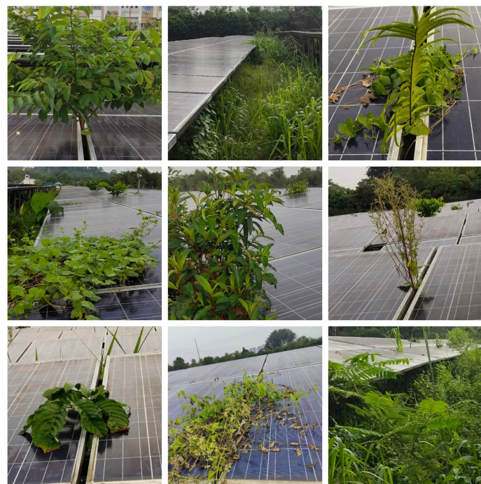
Figure 4. Actual snapshots of various weeds leading to permanent shading of the PV.
