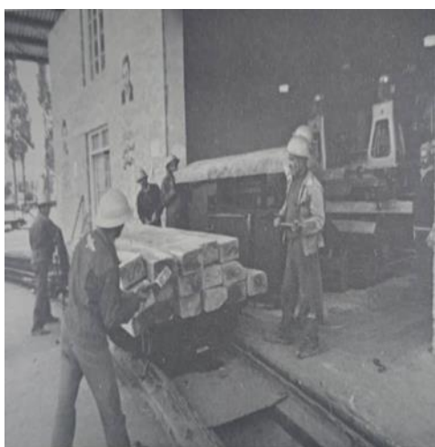
Fig. 1: Preparing railway sleeper in Shirgah plant (1932)
