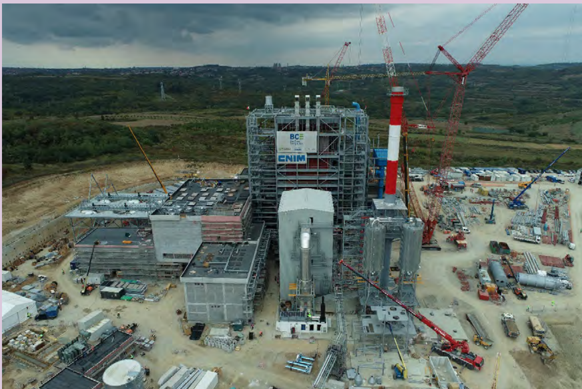
Work in progress on the Vinča landfill, June 2021. Photo credit: Beo Čista Energija
