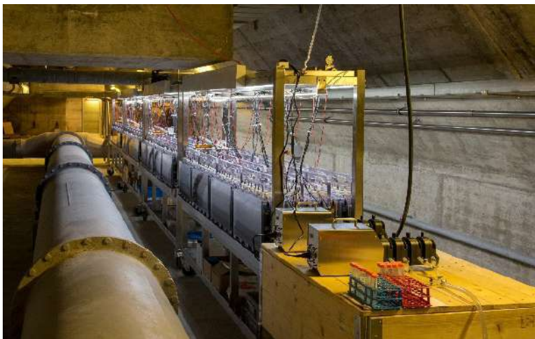
Fig. 1: 1000-L Microbial fuel cell in Wastewater Treatment Plant
