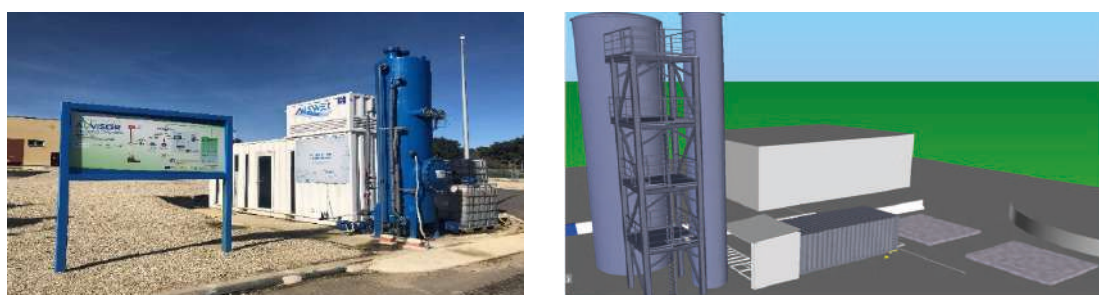
Fig. 1. Demo-scale plant in Guijuelo (left) and 3D model of the demonstration WWTP based on ELSAR™ (right).
