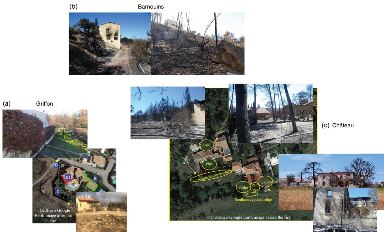
Fig. 3. Pictures of post-fire damage recorded in the three study cases. (a) Griffon (A1, damaged house; B, undamaged house; C, hedge impacted by the residues left on site; D, hedge impacted by the fire front), (b) Barnouins and (c) Château.
