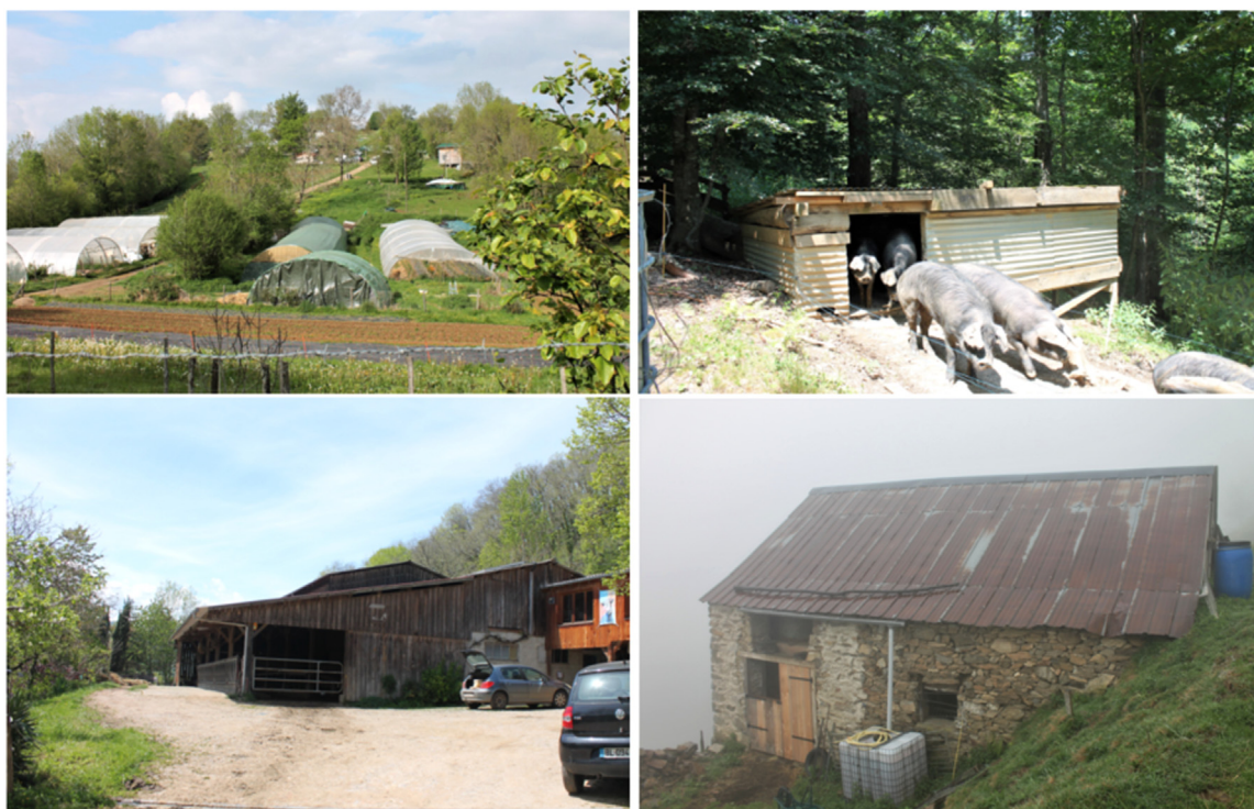
Fig. 8. Production buildings for storage (crops, fodder, tools, etc.), animal stabling and cultivation. Tunnel greenhouses are mainly used for market gardening (photo 1, Ariège), and also sometimes for stabling animals in more progressive farms. The practice of self-construction and the use of wood are also widespread, as shown in photo 2 (pig shed made of wood and reused corrugated steel sheets, Ariège) and photo 3 (3-in-1 building: stabling/storage/milking parlour, Ariège). Buildings can be refurbished also to be used to stable animals, often as a forced choice, while waiting to obtain funds to invest in a new and more functional building (photo 4: traditional sheep pen, Ariège). Photo credit: O.R., 2022.
