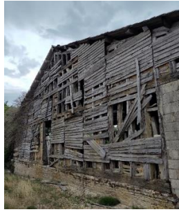
Fig. 1 : West façade of a house built with timber-framing and wattle and daub filling, covered with "tavillons", in Frampas, Champagne, France.
