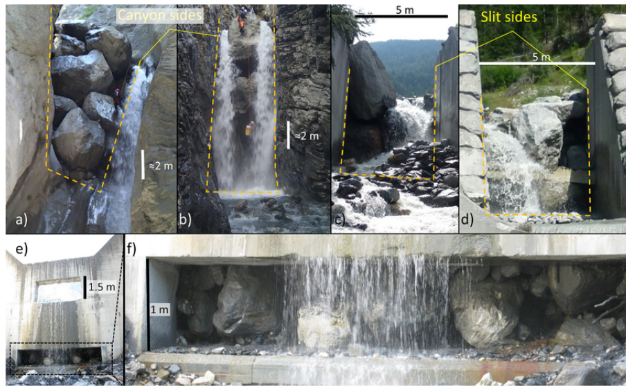
Figure 1: Examples of boulder jamming from debris flows in the French Alps. Figure taken from Piton et al. (2022).
