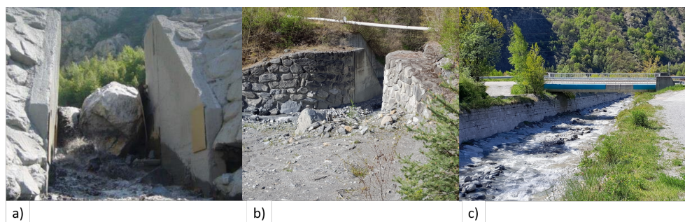
Figure 4: Constrictions within the alluvial fan of the Torrent du Saint-Martin included in the model. The Upper Debris Basin is shown in panel a), the Lower Debris Basin in panel b), and the Upper Bridge in panel c). Photos from Carlados et al., 2022.
