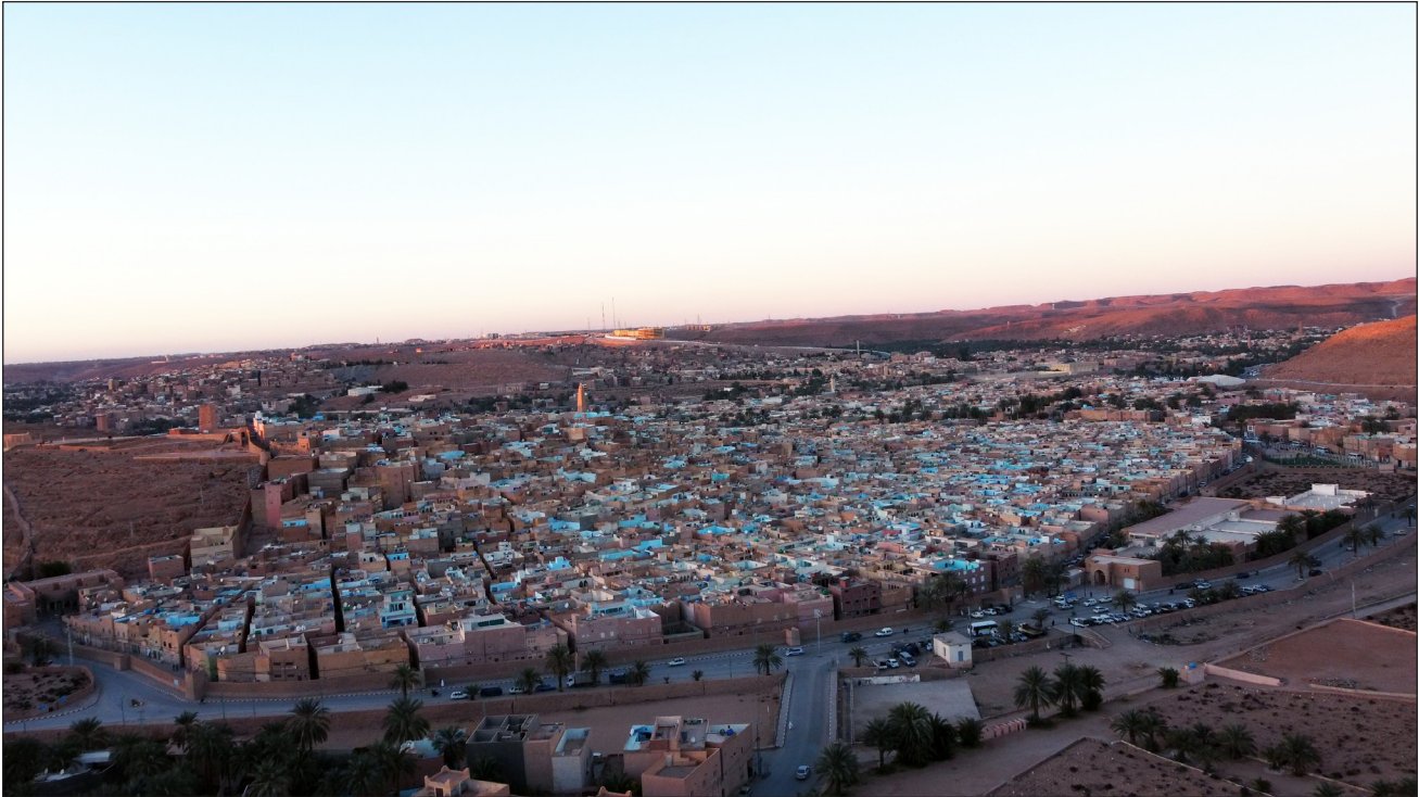
Figure 2 Beni Isguen fortified village (Ksar) from the sky (source: M Khoudja, July 2023).
