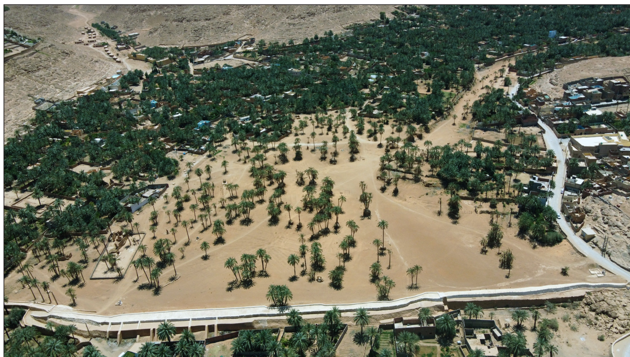
Figure 6 Traditional dam (Ahbass) view from the sky (source: M Khoudja, July 2023).
