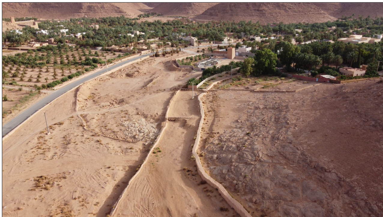
Figure 4 Bouguefa wall diverting water from the Wadi N'Tissa to the palm grove from the sky (source: M Khouadja, July 2023).
