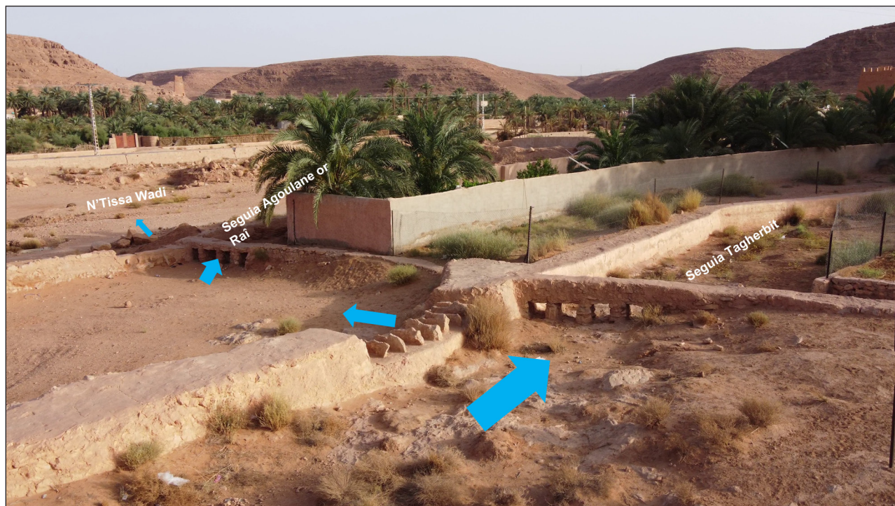
Figure 5 Space for sharing and controlling the water flow at The Beni Isguen palm grove entrance from the sky (source: M Khouadja, July 2023).
