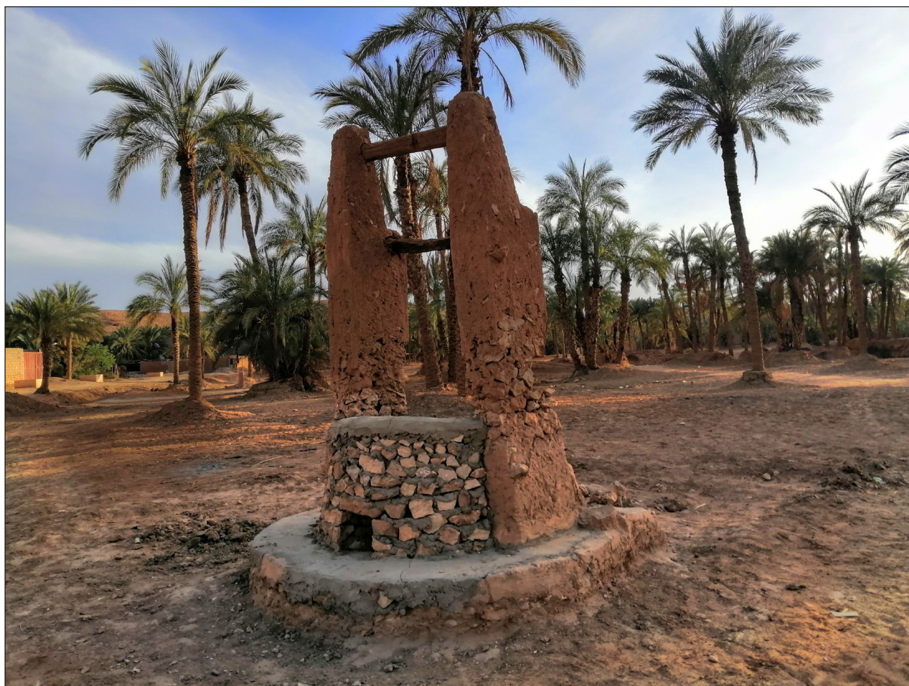
Figure 7 Recharge well restored during the national lockdown period in 2020 (source: M-A SAIDANI).
