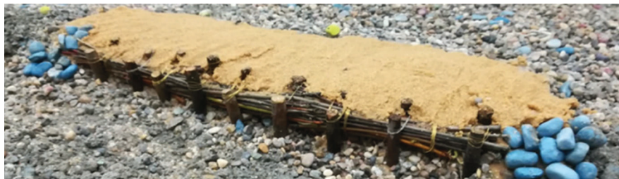
Fig.2A fascine with ripraps upstream and downstream
