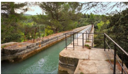
An irrigation canal in southeastern France.
