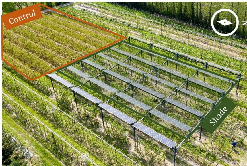
Figure 1. View of the dynamic agrivoltaic system in the apple orchard constructed by Sun'Agri in Mallemort (France).
