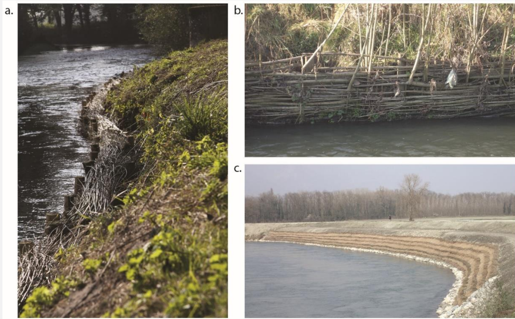
49 Figure 1: photographs of bank protection structures based on SWBE: (a) a living fascine; (b) a living 50 wattle fence; and (c) brush layers above riprap
