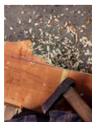
Fig. 5: hewing the edge of a board, photo by the author.
