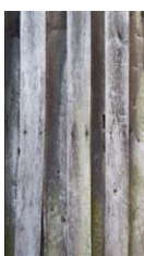
Fig. 2: boards on boards on an outhouse, Västra Götaland. Photo by the author.
