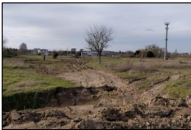
Figure 44. Trenches dug in La Bouillie to prevent illegal settlement. Source: Cardinal (2022).
