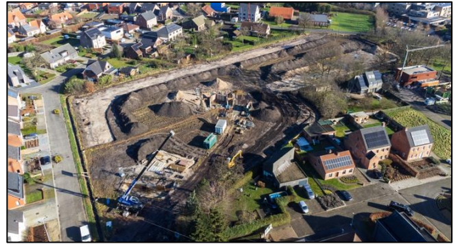
Figure 9. Construction of the flood retention area. Source: Province of Antwerp.
