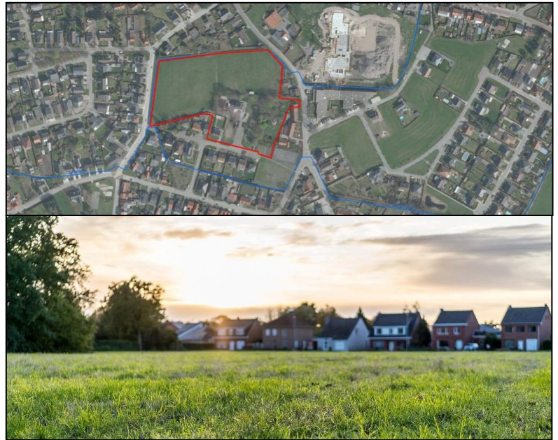
Figure 8. The area that will be transformed into a flood control area. Source: Dienst Integraal Waterbeleid, Provincie Antwerpen.
