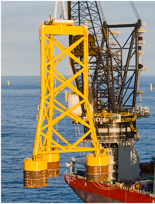
Fig. 1. Multi-bucket jacket foundation at the Borkum Riffgrund 2 installation (image gently provided by NGI/Ørsted).
