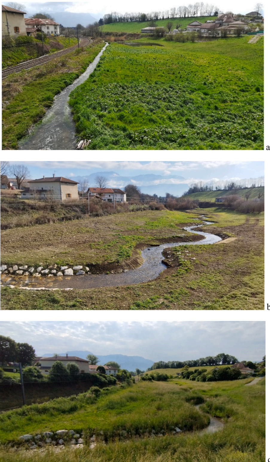
Fig. 2. Restoration of a degraded stream through meanders, in 2021 (a), 2022 (b) and 2023 (c) (Olon River, France; pictures by F. Rey).
