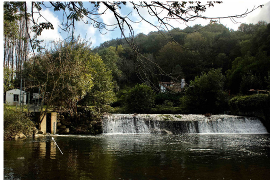
(b) Uxondoa dam with the entry of the fish pass at the left (white arrow)
