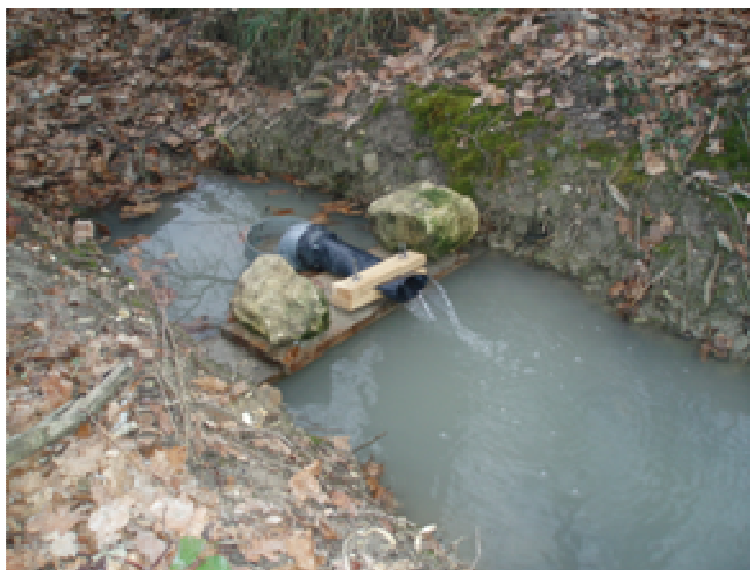
Fig. III-14: Inlet controlled section to maintain a 0.3-L/s flow rate.
