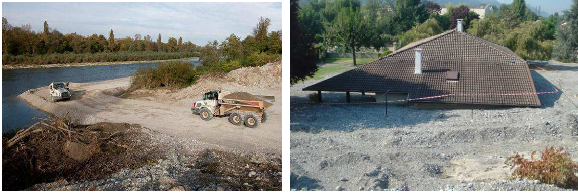
Figure 1: (a) Injection of 25000m 3 of sediments for ecological restoration of the Rhine River near Kemb (photo Alsace.fr) (b) Sediment deposition on the Domenon River and its impacts on population safety (Photo Belleudy)
