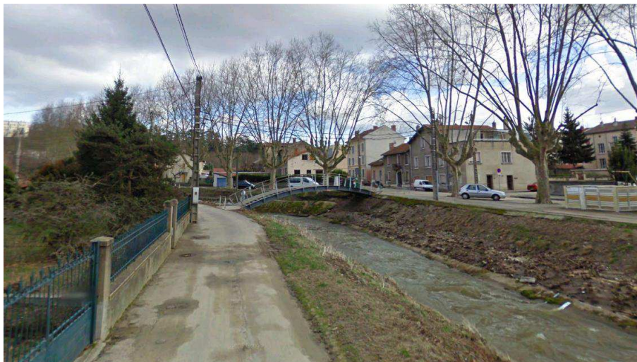
Figure 6.16 : Small bridge at stage gauge L_2 location photographed after the 2009 flood (Source: Google Map)
