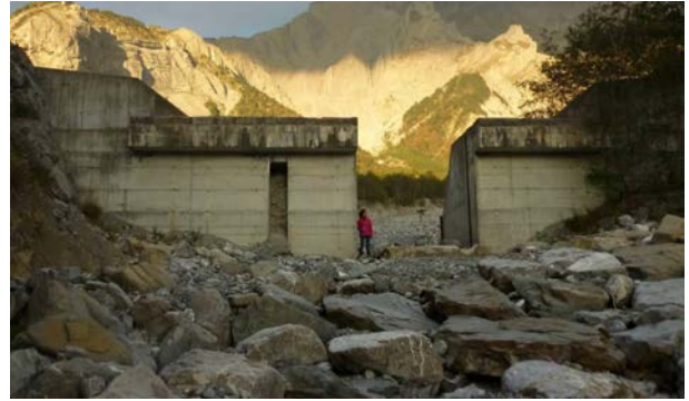
Figure 2.10 – Downstream view of the slit dam on the Ebron torrent (Tréminis (38), FRA), the initially triple small slit dam built in 1990 (see one obstructed slit on the left) has been cut ca. 1998 to become a large slit dam. This operation having deteriorated the structure strength, a big rip-rap layer fixed with concrete has been added on the dam upstream side to increase the structural resistance to debris flow impact. (image by Guillaume Piton)
