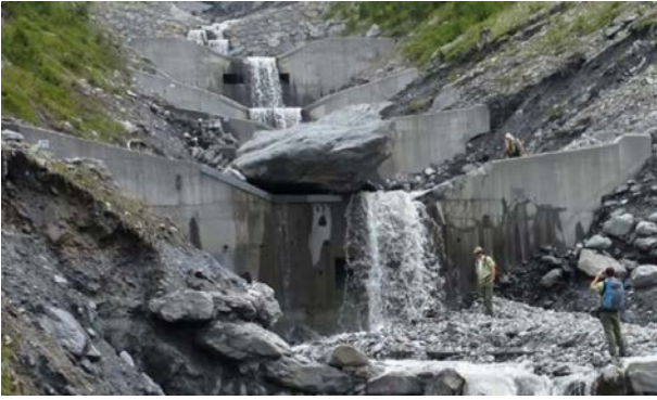
Figure 1.9 – Huge boulder stopped on the check dam series of the St. Antoine torrent upper basin (73 – FRA.) – 2014 (photo courtesy of S. Carladous)
