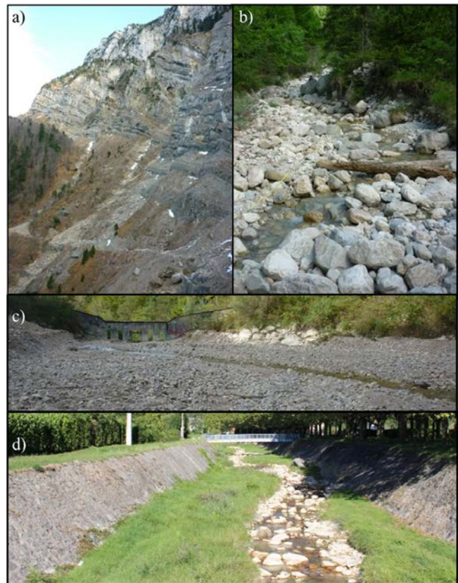
Figure 4.3 – Pictures of the Roize catchment: a) headwaters: marl-limestone cliffs drained by check dam-equipped steep channels; b) coarse Roize bed at the measurement reach c) sediment trap and its open check dam and d) trained fan channel experiencing weak sediment transport as demonstrated by the well-developed grass (Photos by Guillaume PITON)
