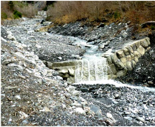
Figure 5.1 – Check dam series in the Saint Julien Torrent (73) Fr – 2015, grade control structure built above the bed level (photo courtesy of S. MEJEAN)
