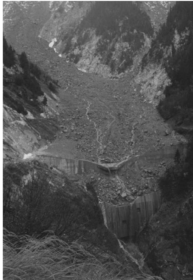
Figure 1.7 – Bon Attrait deepseated landslide and its double consolidation dam ( \approx 100m wide, from left to right bank wings), Ravoire de Pontamafrey torrent (73) Fr., construction: 1968-1970 (photo Nov. 1979 by JL. Boisset courtesy of ONF-service RTM 73)
