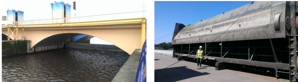
Figure 6.3: Pictures of a shutter in operation (left) and a shutter and upper gate taken out of the dam for maintenance (right).
