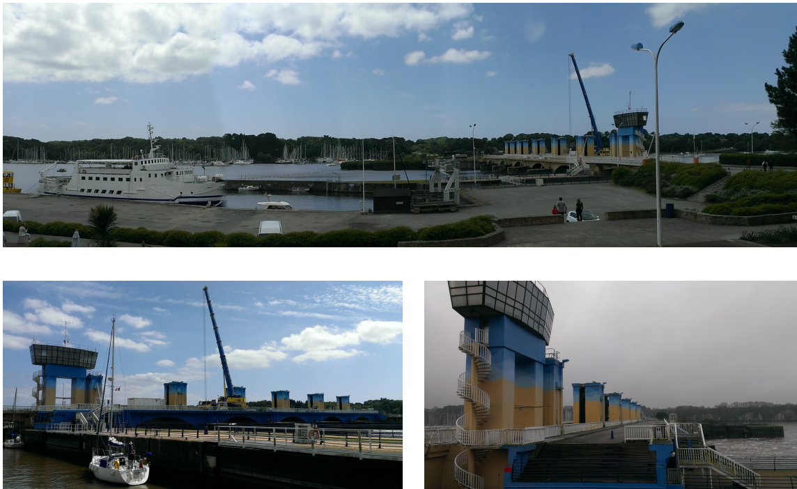
Figure 6.1: The Arzal dam seen from upstream (top), from downstream with the lock in the foreground (bottom left) and from downstream with a lateral view of the dam (bottom right).
