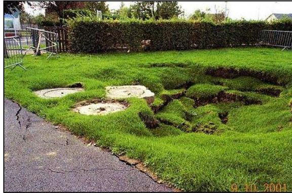
FIGURE I-12: PHOTO D'UN EFFONDREMENT EN SEINE-MARITIME EN 2001 (SOURCE: CETE NC)
