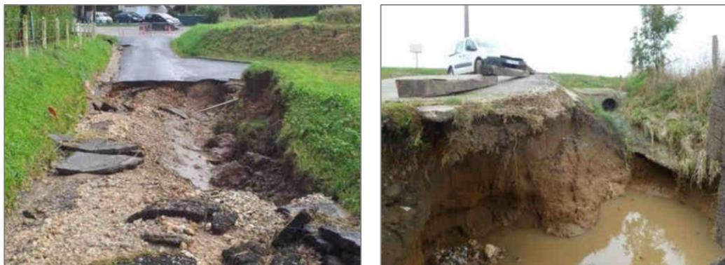
**FIGURE II-3: PHOTOS DE ROUTES EN CAVEES IMPACTEES LORS D'UN EPISODE DE RUISSELLEMENT INTENSE SUR LE BASSIN VERSANT DE LA LEZARDE EN OCTOBRE 2013 (SOURCE : SYNDICAT MIXTE DE BASSIN VERSANT - SMBV - POINTE DE CAUX)**
