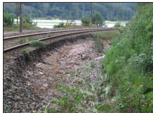
FIGURE I-45: EMPOTEMENT LONGITUDINAL DE BALLAST PAR CIRCULATION D'EAU AU NIVEAU DE LA PISTE OU DU FOSSE
