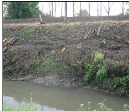
**FIGURE I-52: AFFOUILLEMENT DU PIED DE REMBLAI**
