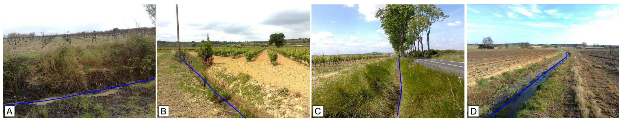
Figure 3.1: Four examples of man-made drainage features in the Hérault département in the south of France: (A) a small ditch conveying runoff at the bottom of a terrace front on a hilly landscape, (B) a ditch in a flat area, (C) a roadside ditch and (D) a sunken path that also acts as a drainage ditch.
