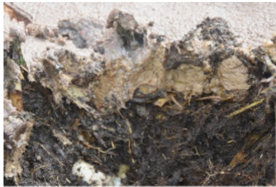
Figure 2.47: Clogging layer (light brown) over a surface deposit layer (dark brown) in a mature French VFTW.
