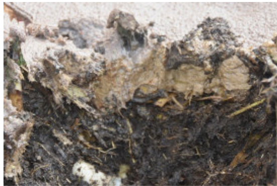
Figure 2.47: Clogging layer (light brown) over a surface deposit layer (dark brown) in a mature French VFTW.
