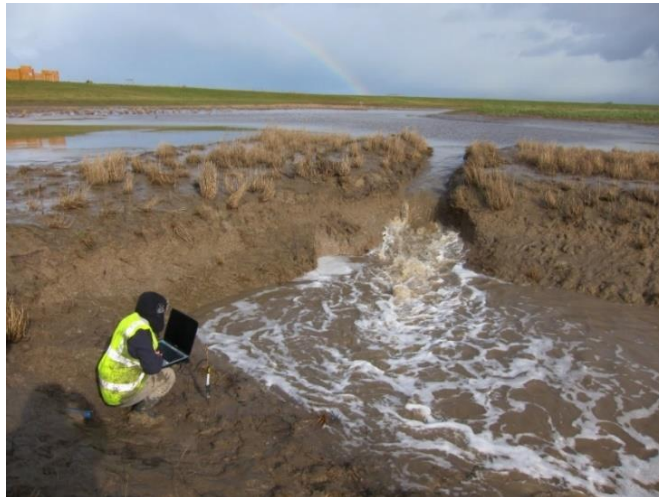
Figure 8.5: Ebb flow routing through pre-excavated channel head tributary at Steart (Photo taken by Anas Anuar, 23/02/2015). This has continued to expand, leading to secondary channel formation into the adjacent marsh.
